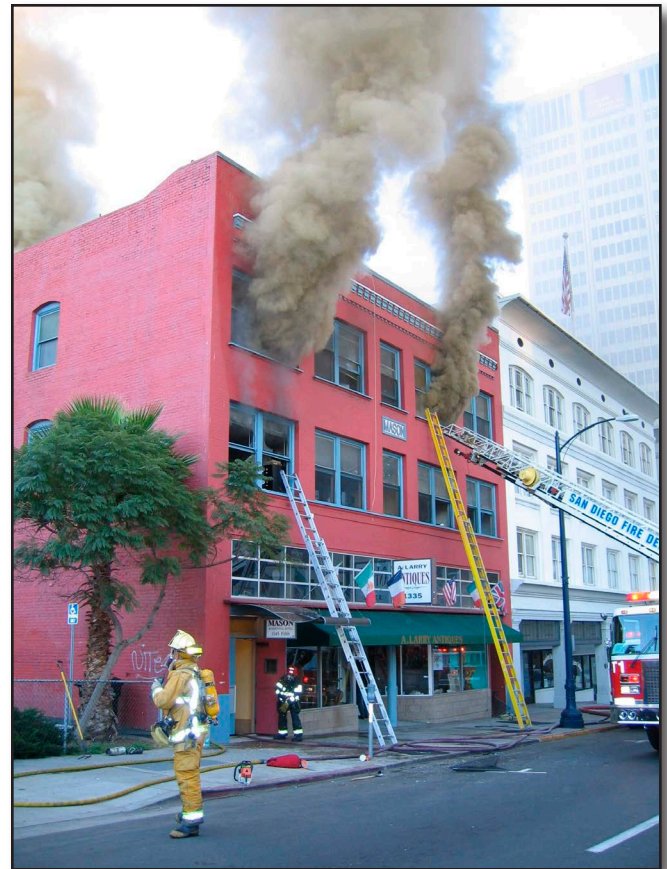
Figure 20-21 Positive Pressure Ventilation in multistory buildings must be a well coordinated and planned event.
