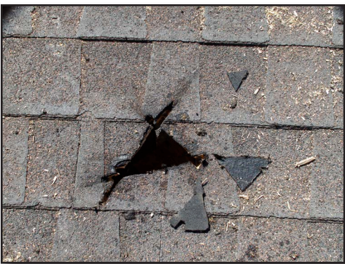
Figure 20-11 Smoke Indicator Hole
