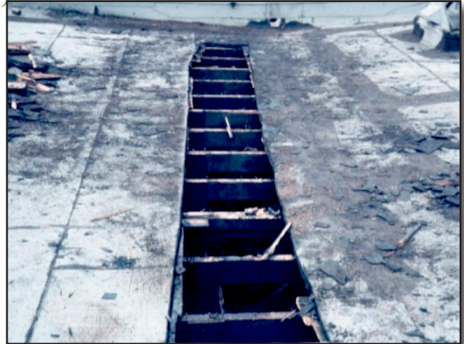
Figure 20-5 Trench (Strip) Cut - Defensive Tactic
